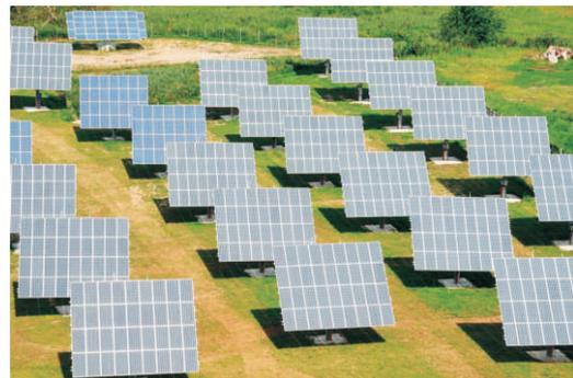
630 kW tracking system in Sluneta-Dobruy, Czech Republic
