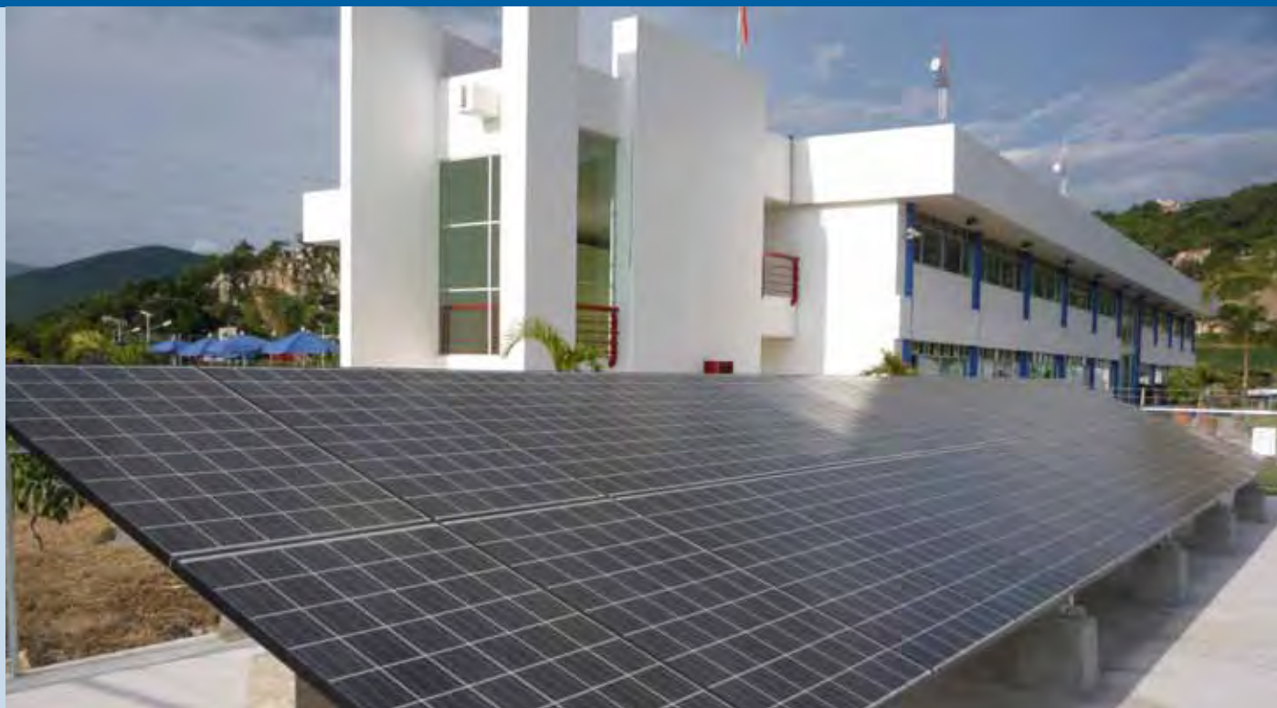
Fig. 1 - 6,5 kWp PV Grid-Connected system at the Technological University of Morelos (photo: UTM).
