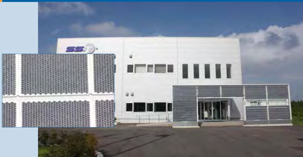
Fig. 3 - Solar Silicon Technology Kazusa Solar Factory PV system, 20 kW (Kazusa-Kamatari, Kisarazu City, Chiba).
