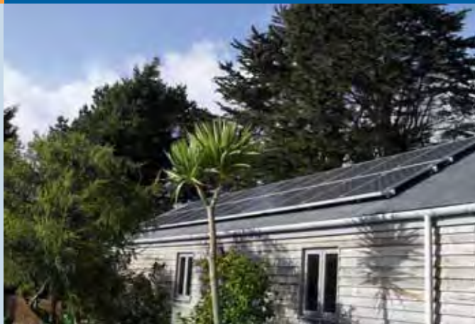
Fig 2 - 4 kWp on a garage slate roof in West Cornwall (photo: Plug into the Sun).
