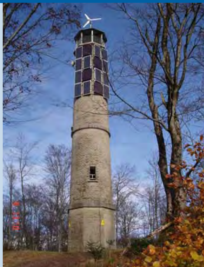
Fig. 3 - Repeater station in the German Black Forest powered by a PV hybrid system (photo: Steca/Fraunhofer ISE - UESP).
