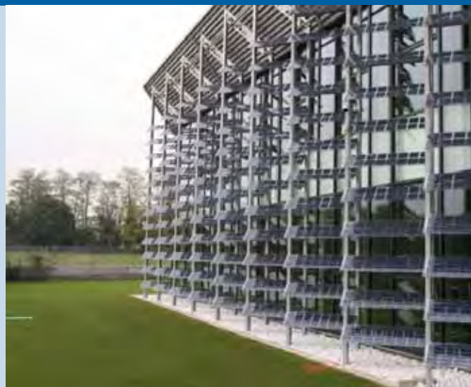
Fig. 1 - 48 kW array mounted on shading elements, Sarcedo (VI).
