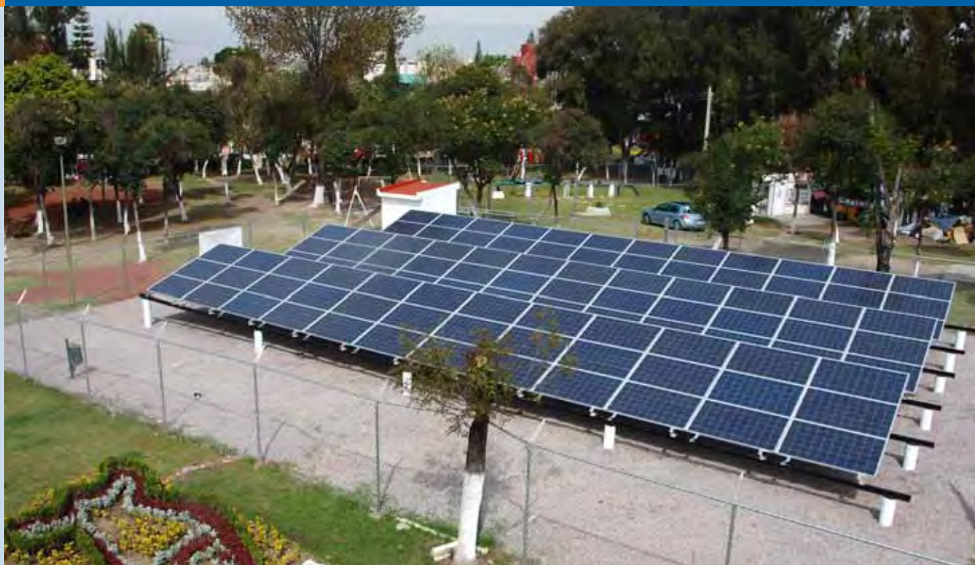
Fig. 4 - 21, 6 kWp Grid Connected System in public park in city of Puebla (photo: Alternativa Energética SA de CV).
