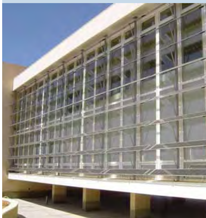
Fig. 5 - PV integration in facade in San Fernando, Cádiz (photo ASIF).
