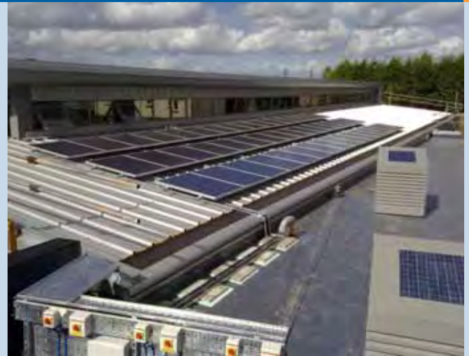
Fig. 5 - 9,7 kWp PV installation - Hamworthy Library, Poole (photo: Sustainable Energy Installations Ltd).
