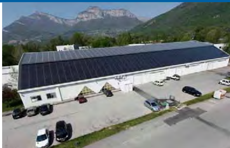
Fig. 1 - PV System on a sport center in Challes les Eaux (Savoie Department) - 203 kW (photo: Edisun Power).
