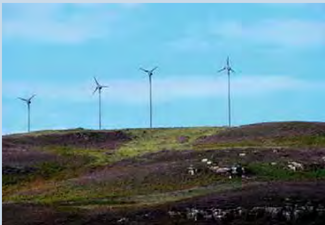
Fig. 1 - The power generation system of the Isle of Eigg, Scotland, consists of 10 kWp PV, 3 hydro plants (100 kW, 2 x 6 kW), 4 Wind turbines (4 x 6 kW) and 2 Diesel gensets (2 x 80 kVA). Each of these sources has been sensitively sited to cause minimum visual and physical impact upon the island's landscape. Twelve Sunny Island 5 kW inverters are used connected in four three phase clusters to provide a total output rating of 60kW. A Multicluster Box enables the communication among the inverters and provides contactors for the connection to the island grid, to the PV and Wind inverters and the back-up gensets. Each cluster is connected to a 48V 2242 Ah (C10) battery bank consisting of 24 batteries. 87 inhabitants owning 37 residential and 5 commercial properties must be supplied by the system. The peak demand has been limited with the approval of the residents; domestic and small business supplies have been restricted at 5kW, and larger business supplies at 10kW.
