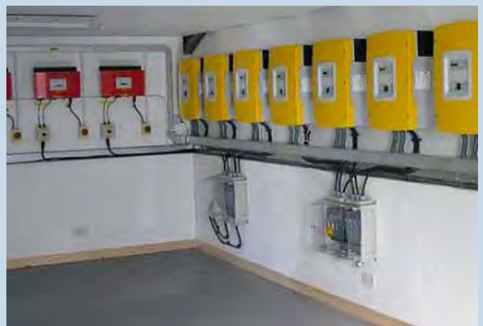
Fig. 1 - The power generation system of the Isle of Eigg, Scotland, consists of 10 kWp PV, 3 hydro plants (100 kW, 2 x 6 kW), 4 Wind turbines (4 x 6 kW) and 2 Diesel gensets (2 x 80 kVA). Each of these sources has been sensitively sited to cause minimum visual and physical impact upon the island's landscape. Twelve Sunny Island 5 kW inverters are used connected in four three phase clusters to provide a total output rating of 60kW. A Multicluster Box enables the communication among the inverters and provides contactors for the connection to the island grid, to the PV and Wind inverters and the back-up gensets. Each cluster is connected to a 48V 2242 Ah (C10) battery bank consisting of 24 batteries. 87 inhabitants owning 37 residential and 5 commercial properties must be supplied by the system. The peak demand has been limited with the approval of the residents; domestic and small business supplies have been restricted at 5kW, and larger business supplies at 10kW.
