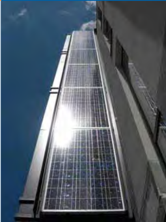
Fig. 4 - 1 kWp PV facade on an Office block in Central London (photo: Bright Green Energy Ltd).
