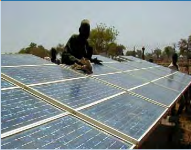
Fig. 3 - Cleaning PV Panels from a solar PV drinking water pumping system in the Sahel - PRS project from the European Commission (photo: IED).
