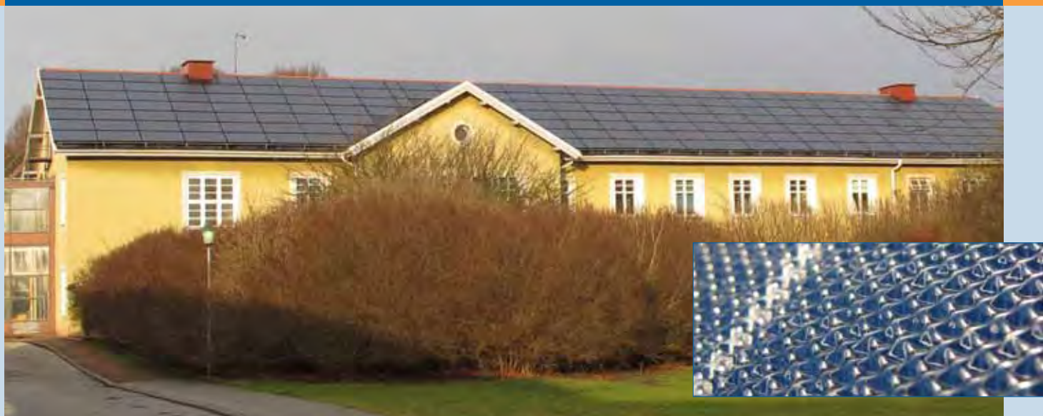
Fig. 2 - 100 kWp of PV modules integrated in the roof of two buildings in Malmö.
