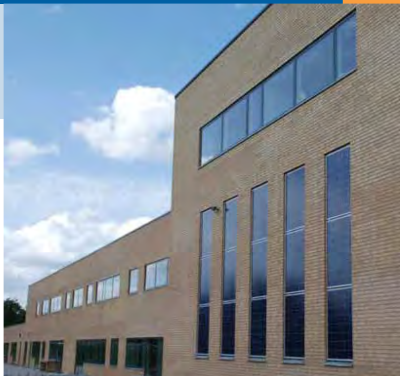
Fig. 2 - School in the Horsens municipality, 2,55 kWp poly crystalline modules integrated in the facades.
