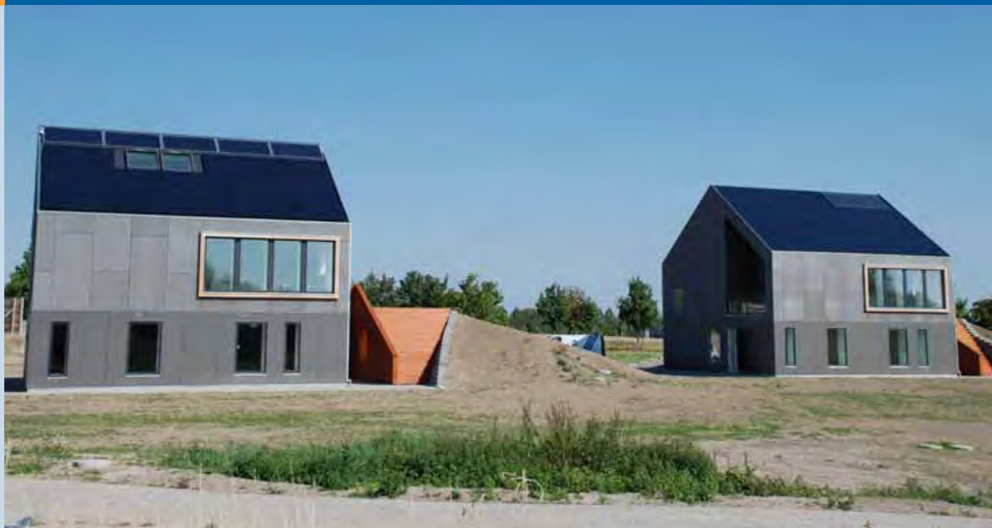
Fig. 3 - Flexhouse at the Danish Technical University, 18 kWp single crystalline modules integrated in the roofs.
