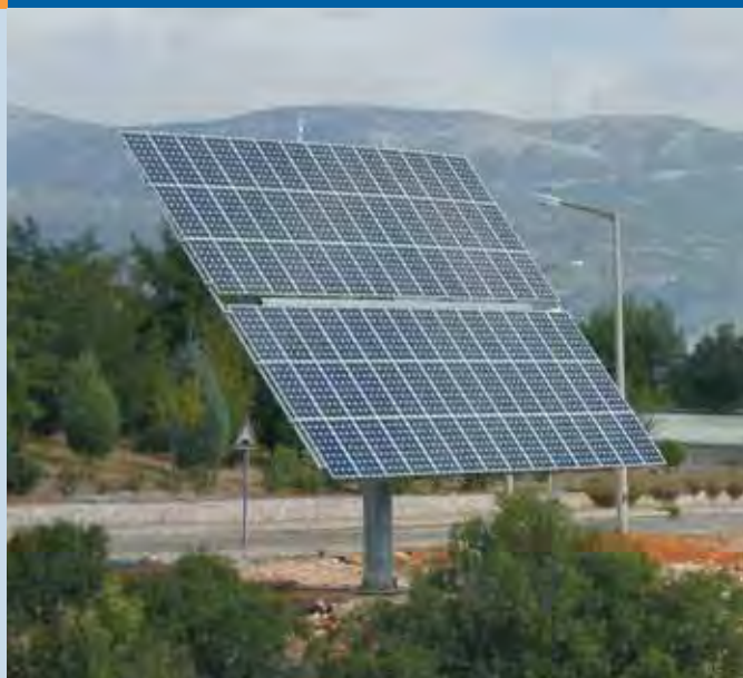
Fig. 3 – 15,6 kWp dual-axis solar tracker PV power system in Mugla, by Mugla University.
